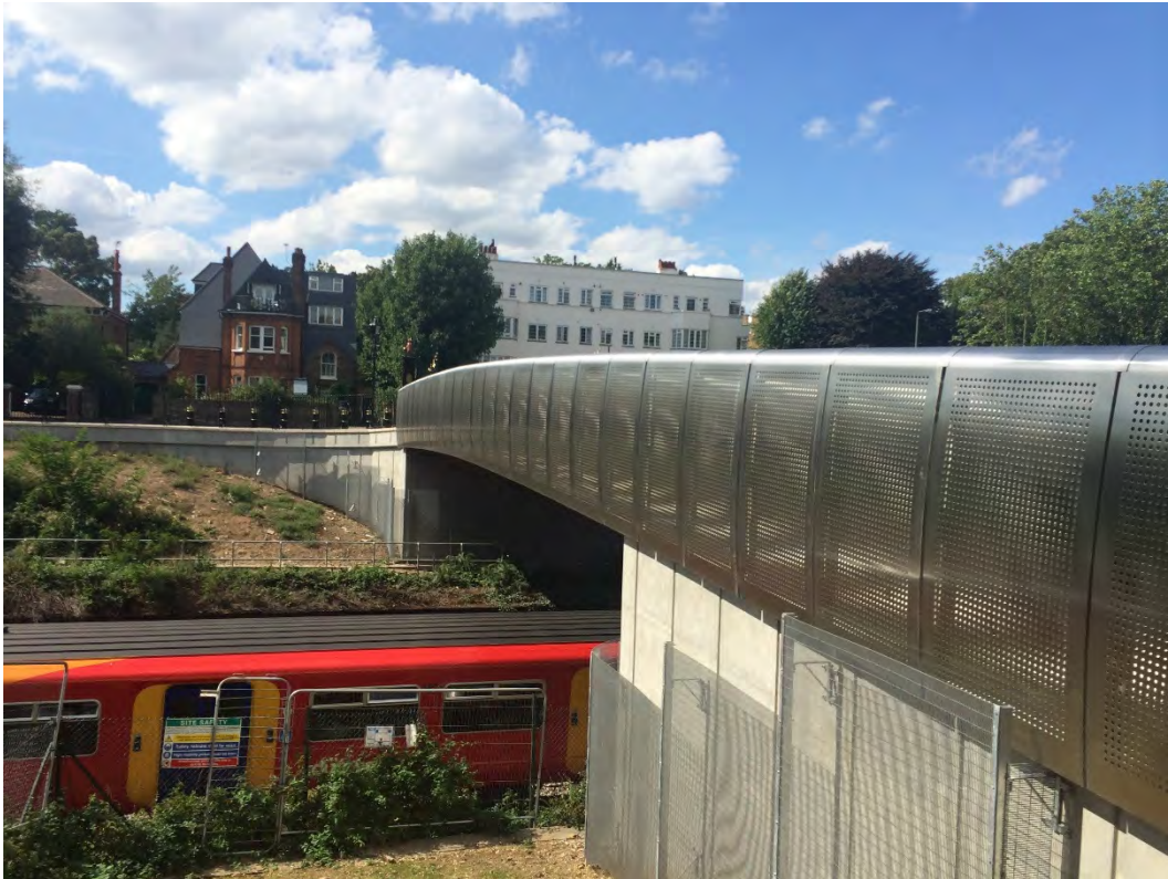
Figure 10: Example Single Span Bridge
